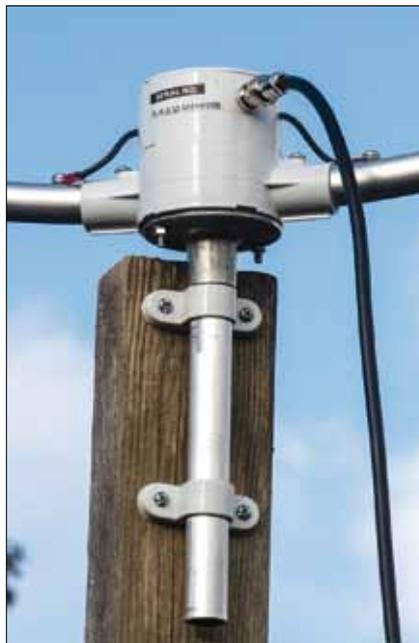
**The ALA1530LN's stub mast mounted on a wooden post using a couple of conduit fixing clips.**
